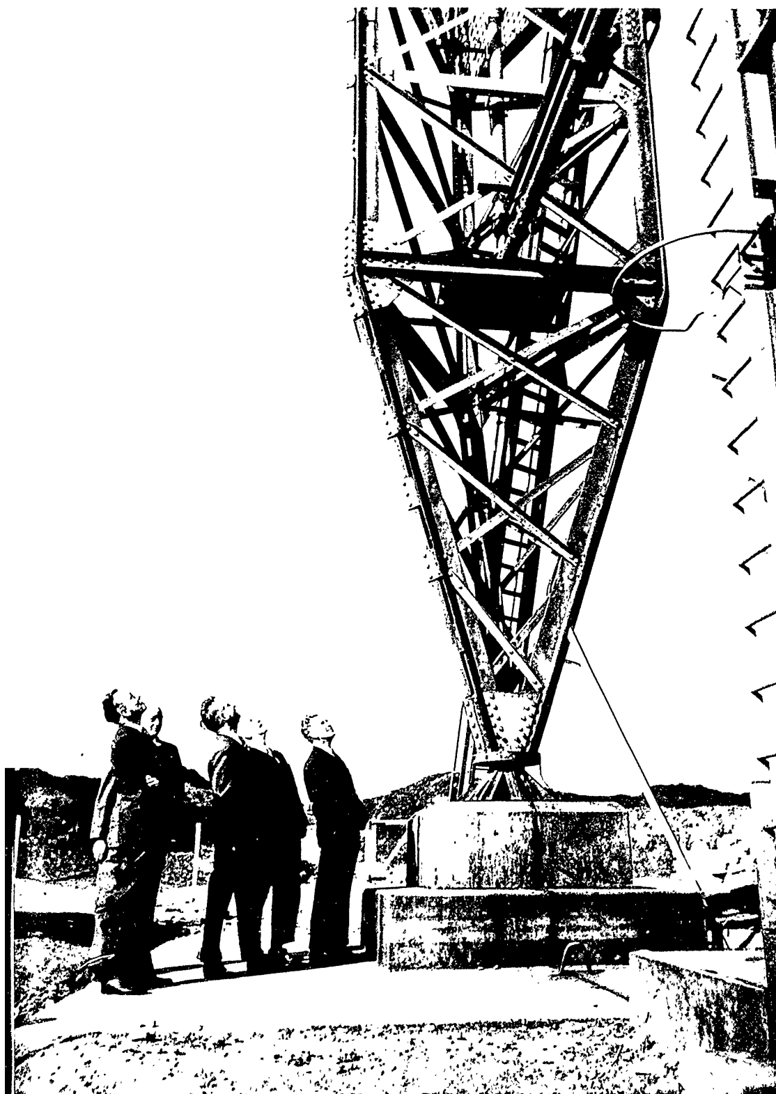
The television transmitting station at Holme Moss was opened in October, 1951. Sir William Haley, then Director-General of the BBC, and members of the Board of Governors take a look at the 750 ft. mast.
