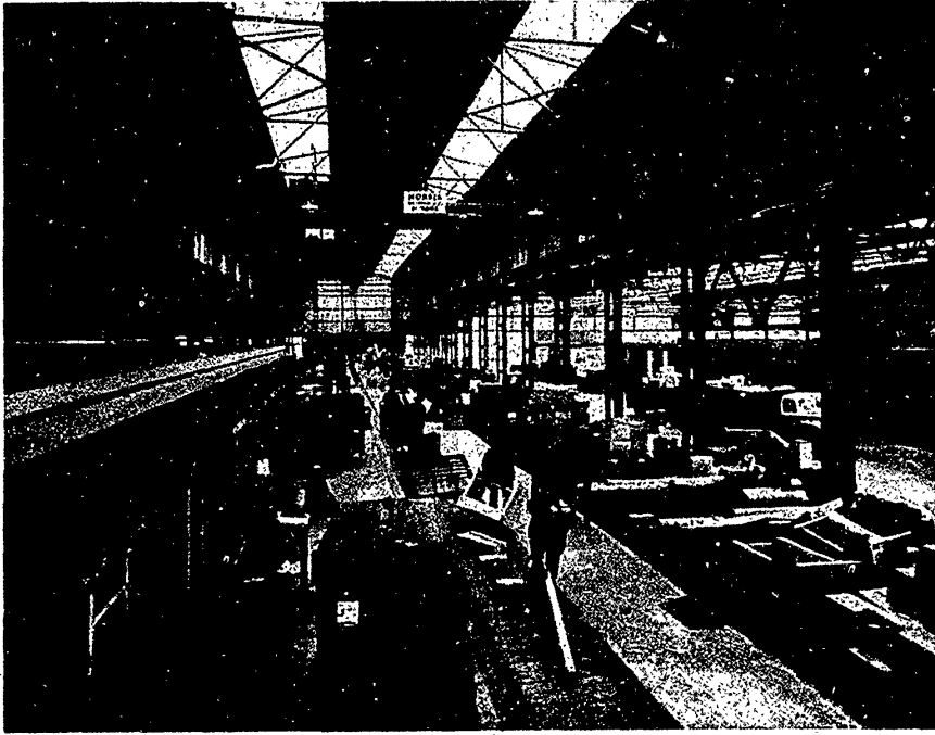
Re-modelled railway freight concentration depot at Walsall which serves 26 towns in an area of 250 square miles.
