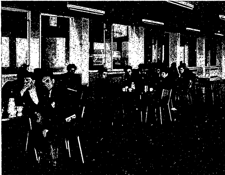
Mess room in new staff amenities block, Bristol (Bath Road) diesel depot.
