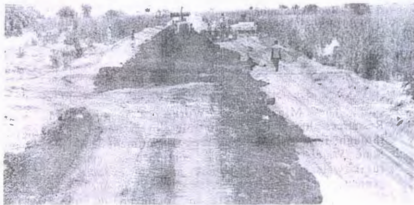
A road under construction
