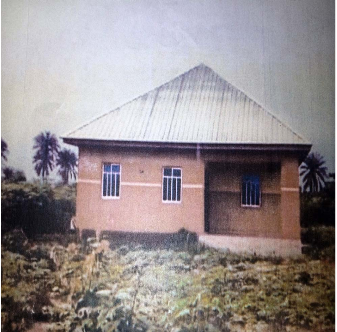
UNCOMPLETED PRIMARY HEALTH CENTRE AT UMUNTEKE, UKWA WEST LGA, ABIA STATE
