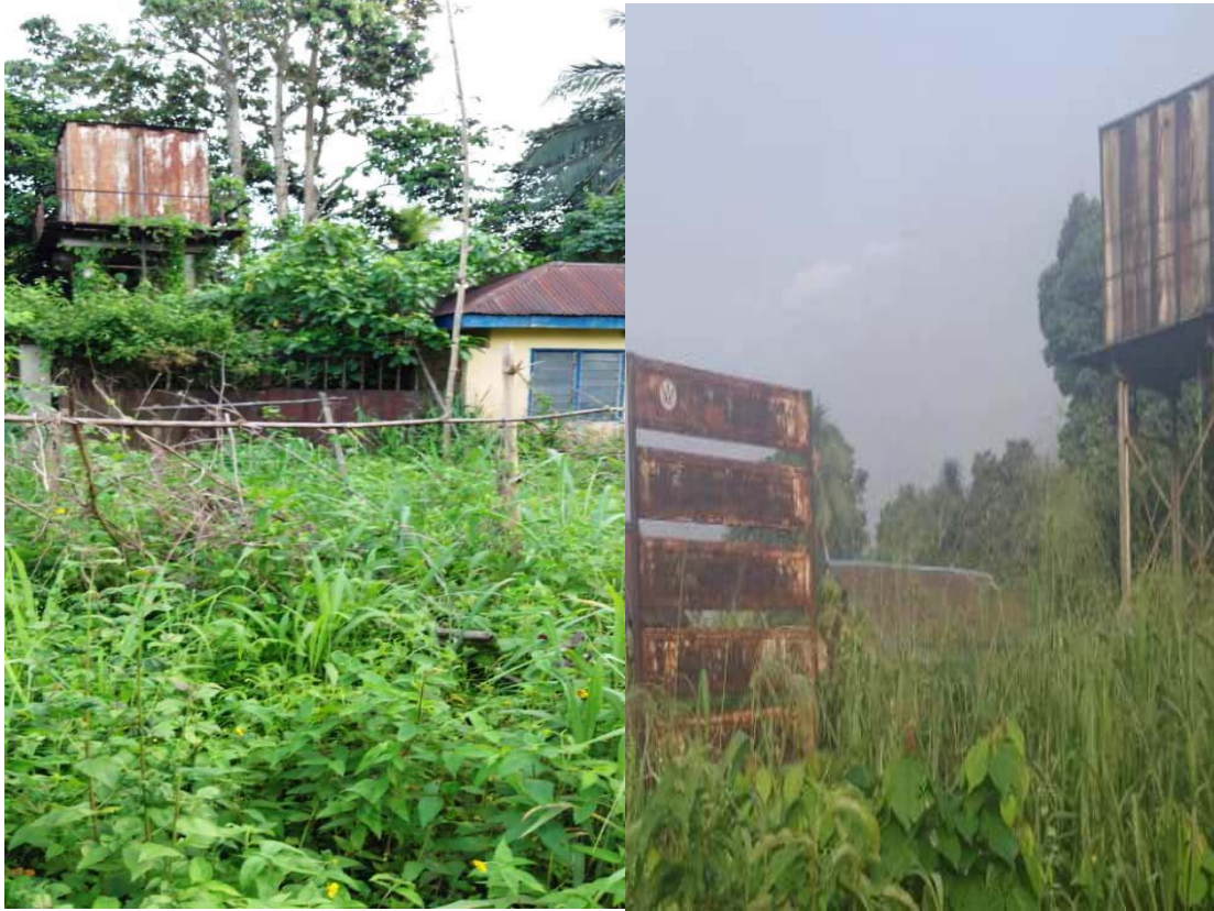
ABANDONED WATER BOREHOLE PROJECTS AT OHURU, UKWA EAST LGA, ABIA STATE
