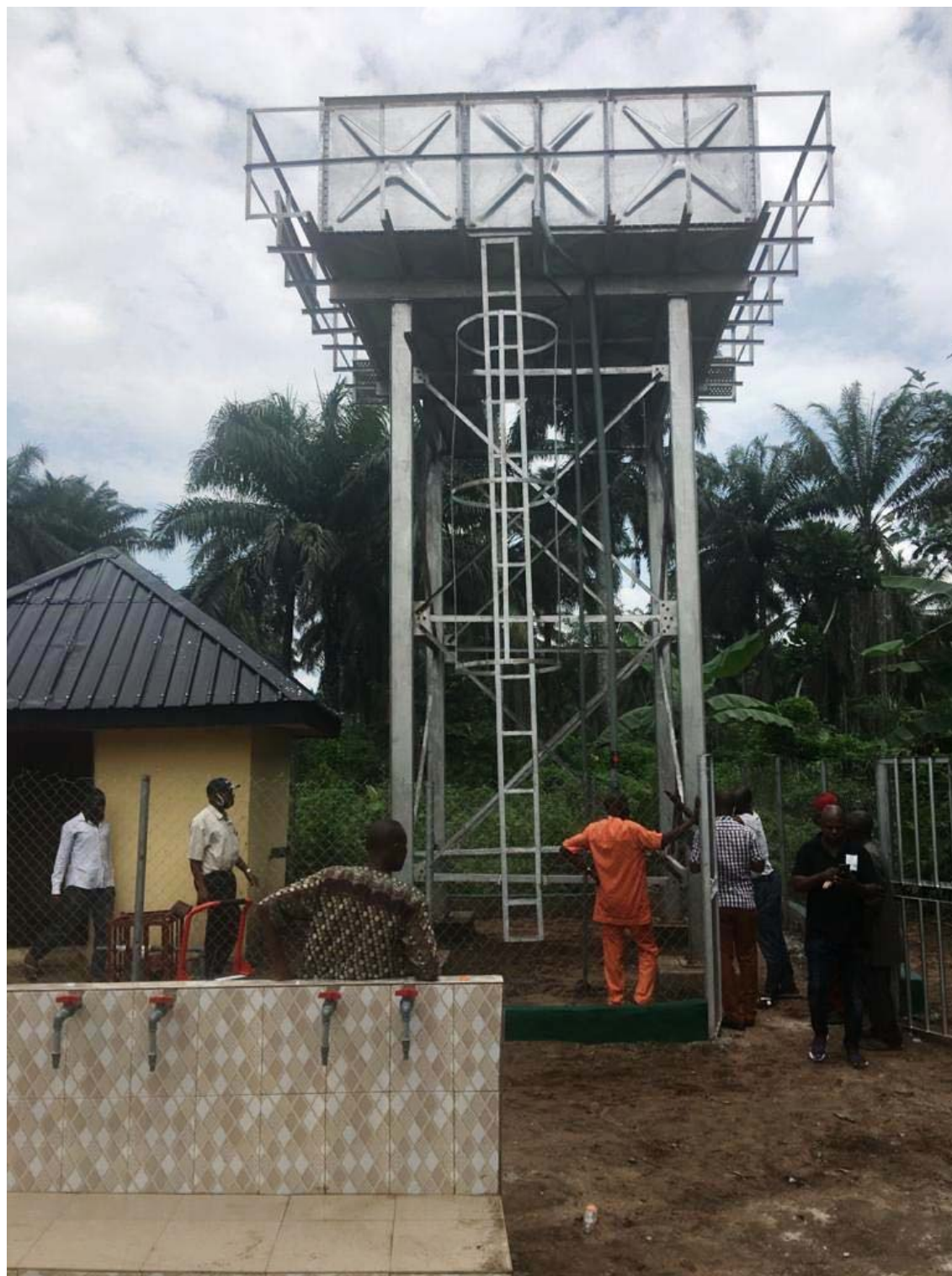
FUNCTIONING WATER BOREHOLE AT OHAMBELE, UKWA EAST LGA, ABIA STATE
