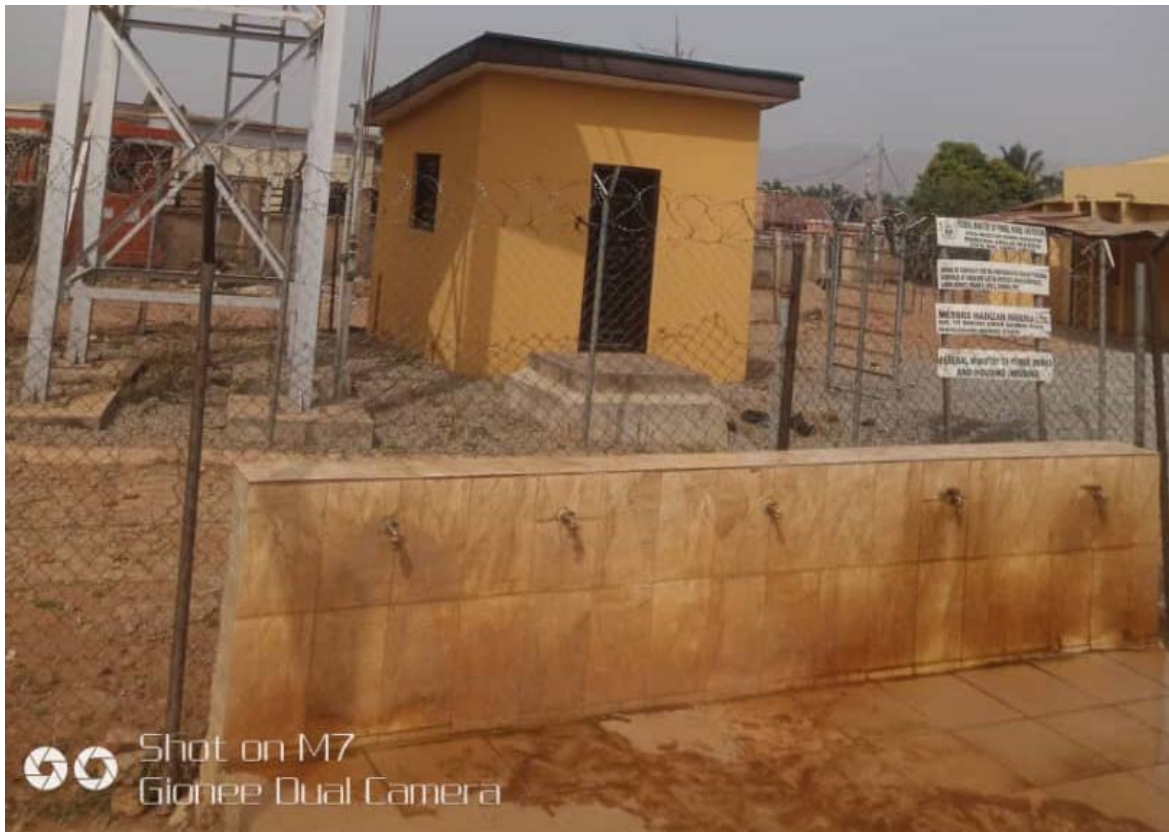
FUNCTIONAL BOREHOLE PROJECT, KUBWA, BWARI AREA COUNCIL
